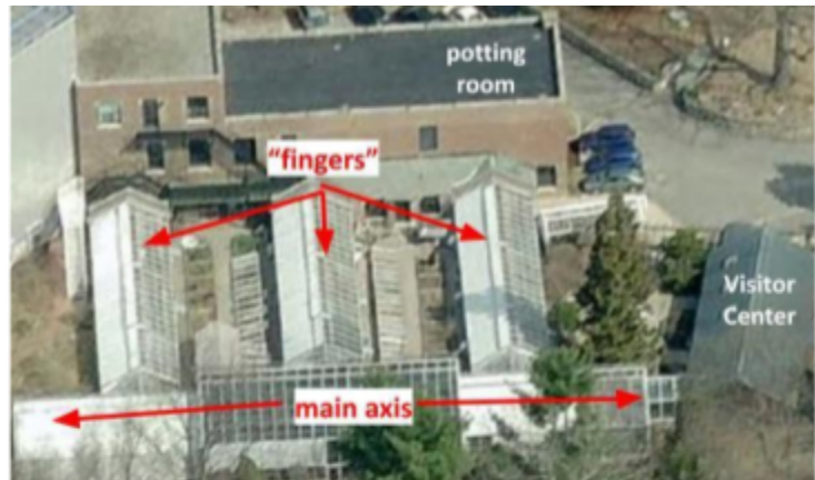
Aerial view of the greenhouses prior to demolition in 2017.
